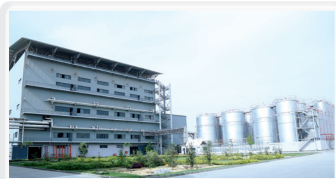
Water Based Emulsion Resins Plant
