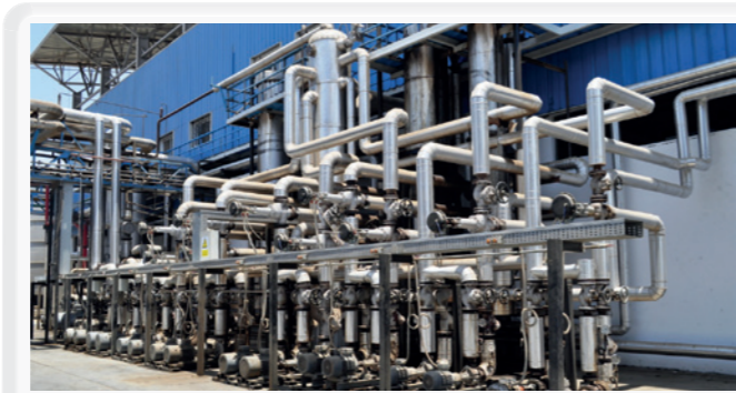
Solvent Based Resins Plant
